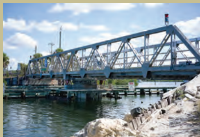
Blackburn Point Swing Bridge Built 1925 Blackburn Point Road, Casey Key, Osprey
