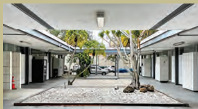
Lawyers Professional Building Built 1961 2051 Main Street, Sarasota Architect, Frank Folsom Smith
